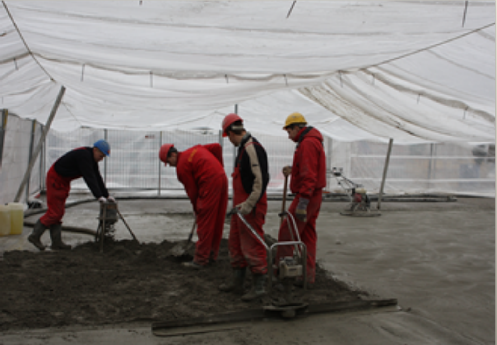
Trowel of PLASTCRETE by skid vibrator to get evenly distributed layer.
