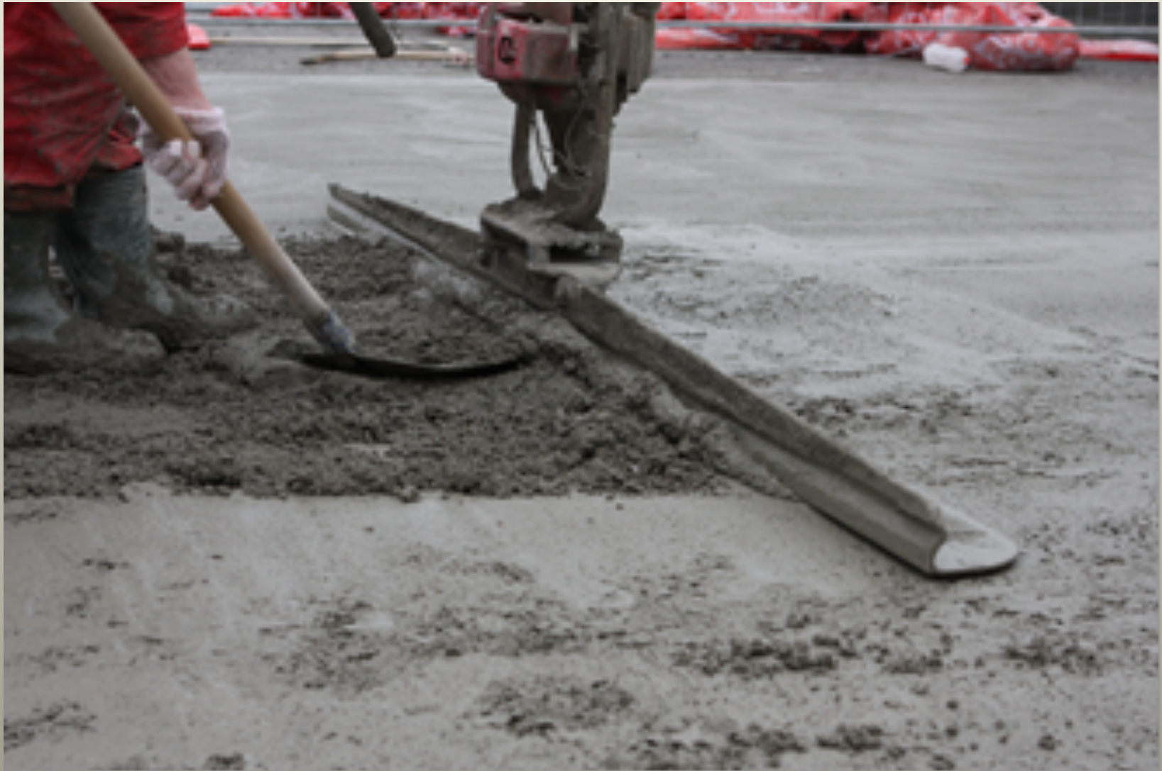
Finishing of PLASTCRETE layer by trowelling with screed vibrator.
