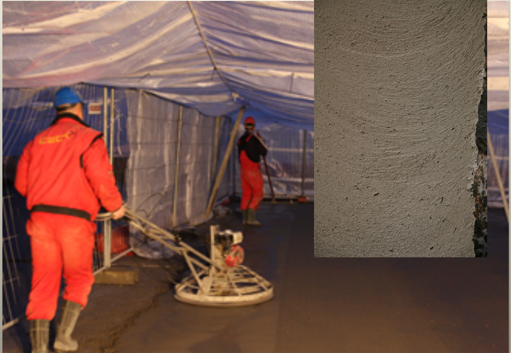
Polishing by the hand operating machine with example of PLASTCRETE surface after first shift (see above at right).
