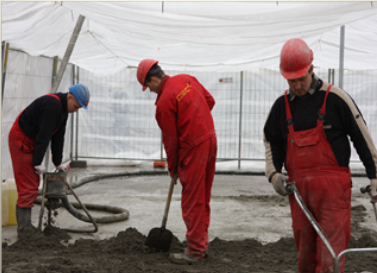
PLASTCRETE batch distribution by the shovels to get 20 mm thick layer.
