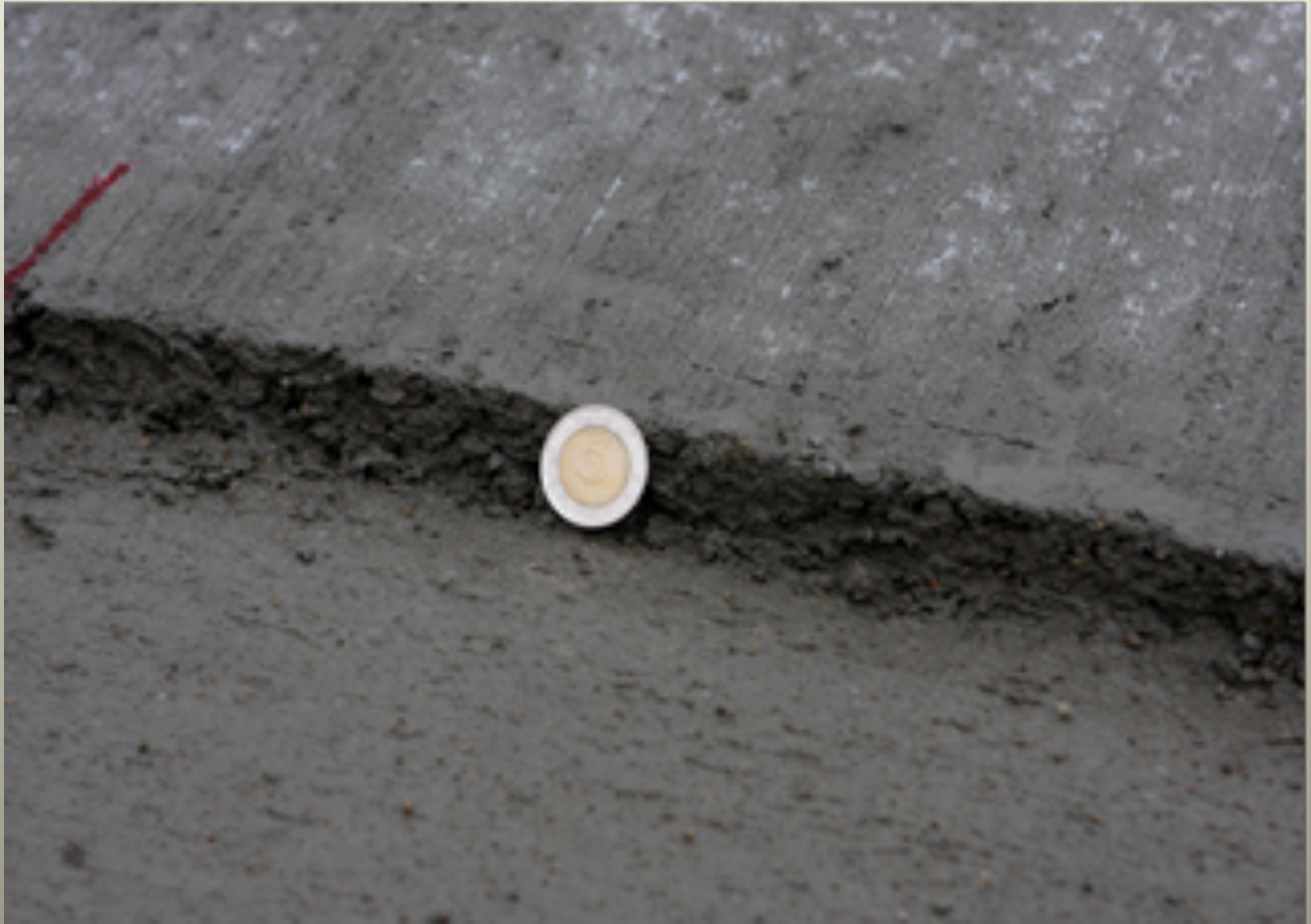
Fresh cut of PLASTCRETE layer is thick at 20 mm before polishing.
